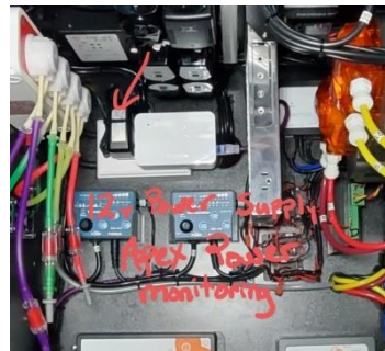
12v Power Supply for Apex Power Monitoring (Inside Cabinet Top Left Corner on Back Wall)
