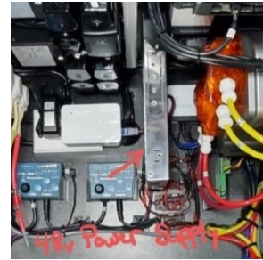
Meanwell LRS-200-48 200W, 48V @ 4.4A (Located Inside Cabinet Under Top)
