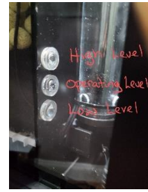
Water Level Sensors (Located in Left Rear Chamber)
